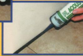
Use 1/2" (13 mm) backer rod and insert it in the 3/8" (9 mm) space. Do the same thing for the obstacles. Apply the acoustic sealer over the backer rod up to the level of the covering. This method give you a better result than the first.
