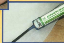
Prepare 7"-wide (178 mm) etafoam strips. Install them before setting the panel on the floor. Then apply an acoustic sealer behind the etafoam up to the covering in order to fill the 3/8" (9 mm) empty space around the room. For the obstacles, fill the empty space with backer rod and apply the acoustic sealer. Or you can simply use the acoustic sealer.
